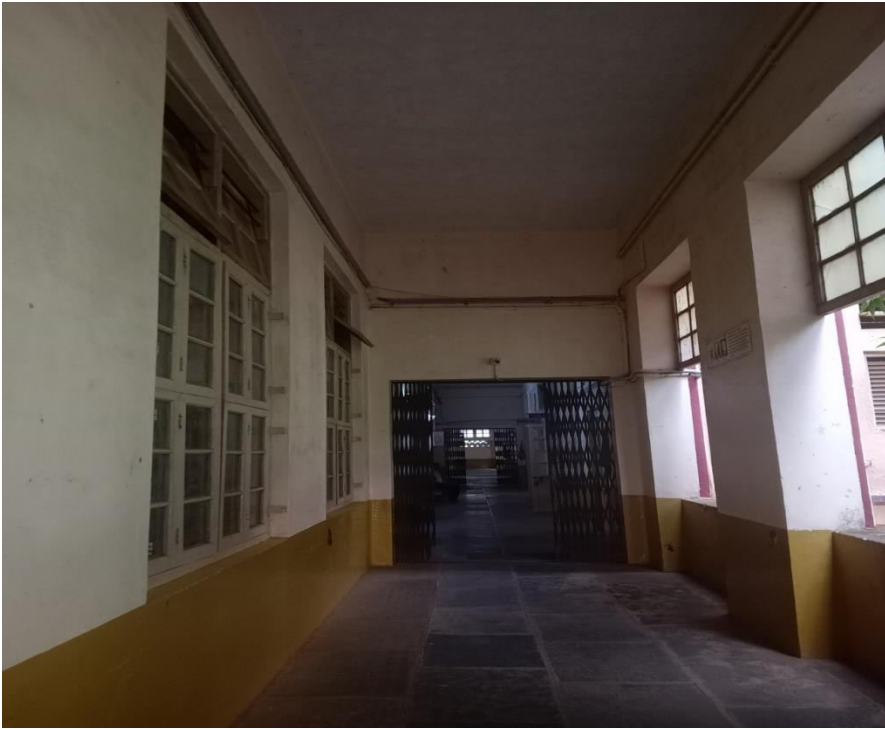
CC-TV Camera surveillance in Physics Department Corridor
